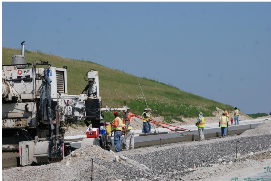
Concrete paving operations near 127 th Street.
