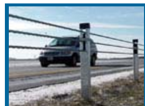
New cable median barrier installed on I-88.
