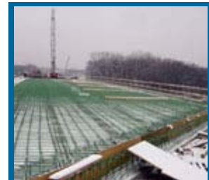
Work continues on bridges south of the Lincoln Oasis.
