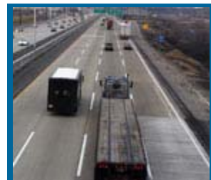
Four lanes now open from Rte. 59 to Washington St.
