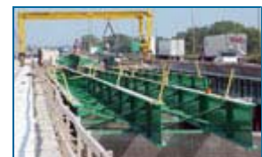
Project includes widening the Markham Yard Bridge.
