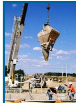
Crews pour concrete for the Cedar Road Bridge over I-80.
