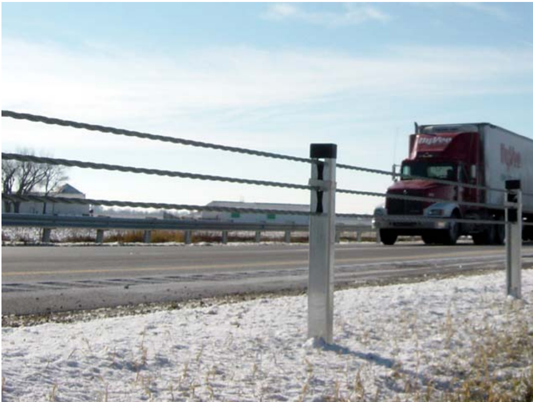
Cable median barriers are in place on I-88 from IL 251 to US 30.
