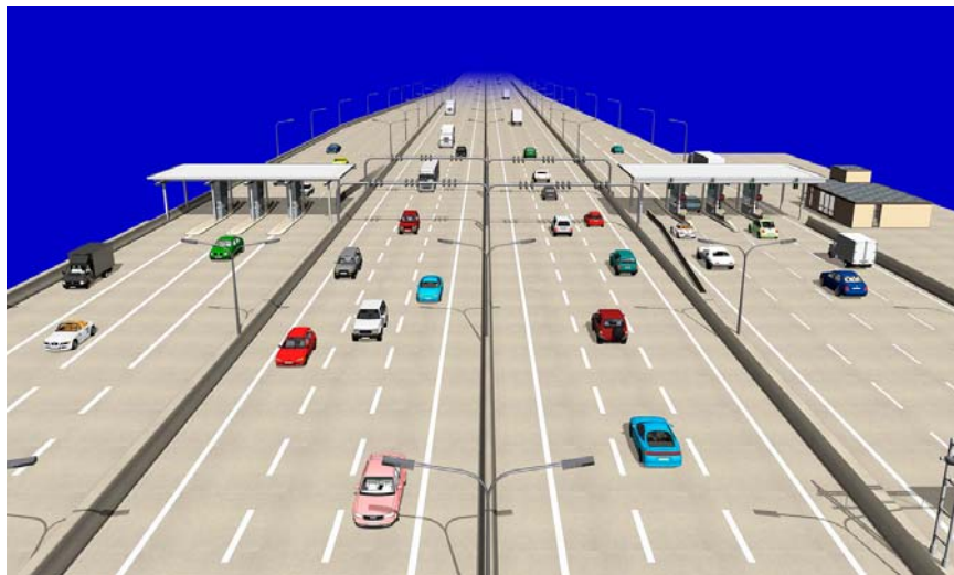
Toll Plaza with Open Road Tolling
