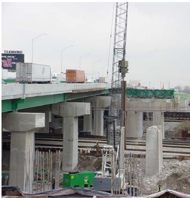
The Markham Yard Bridge was reconstructed and widened.
