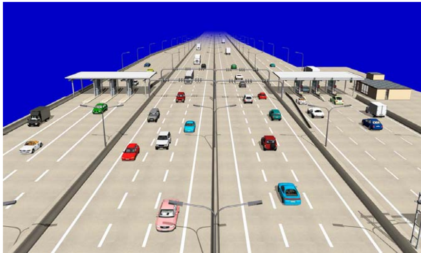
Toll Plaza with Open Road Tolling
