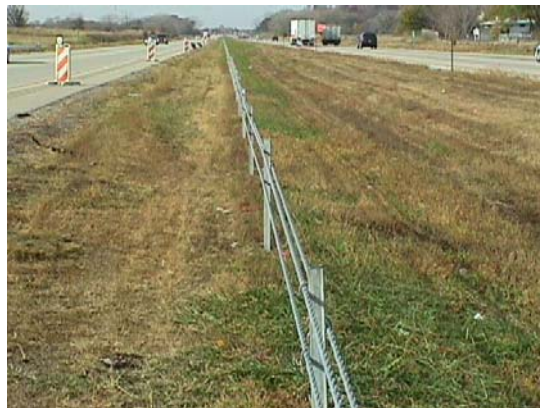
Cable median barrier is now installed on the Northwest Tollway.
