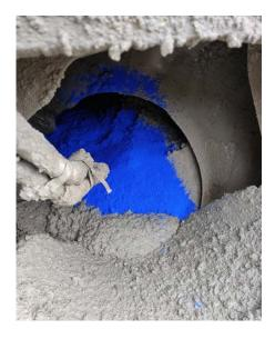
Figure 4-2. Addition of HydroMax
