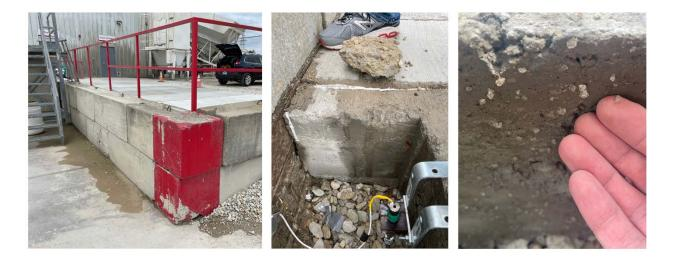
Figure 4-23. Wetness observed around the slabs
