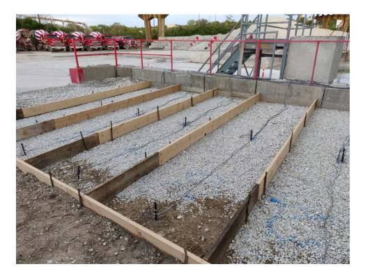
Figure 4-11. Strain gages and positioning chairs setup (photographed facing south)
