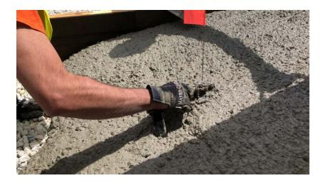
Figure 4-19. Compacting of HPC around the embedded strain gages
