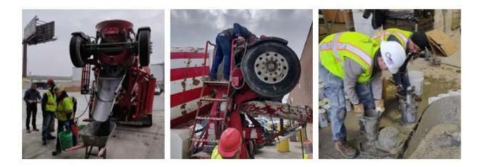
Figure 4-1. Mixing procedure: (left) arrival of mixing truck containing the base HPC mixture, (middle) addition of SAP to back of mixing truck, (right) testing fresh properties and casting cylinders.
