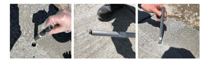
Figure 4-17. Installation of iButtons (L-R: removing plastic pipe after concrete hardened, placing iButton using magnetic stick, covering the space above iButton using the plastic pipe to form a seal)
