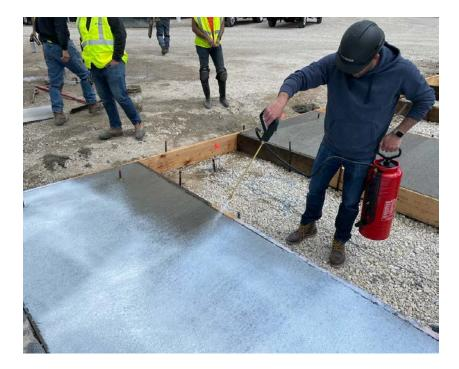
Figure 4-21. Coating the top surface of the HPC slab with curing compound
