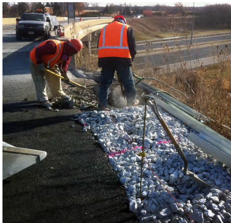
Guardrail installation over the Edens Spur (I-94) near Skokie Boulevard
