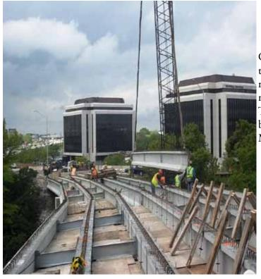
Crews install beams on the Tri-Level Bridge ramp structure from northbound Tri-State Tollway (I-294) to westbound Jane Addams Memorial Tollway (I-90)
