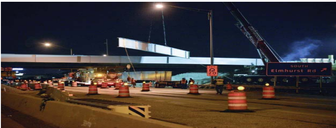
Bridge beams being installed on the new Elmhurst Road Bridge over the Jane Addams Memorial Tollway (I-90).
