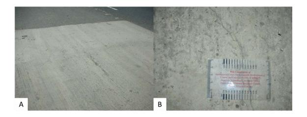
Figure 2-5 – Full-Depth CAC Repair on I-290, Chicago, IL: (A) Overview, (B) Cracking
