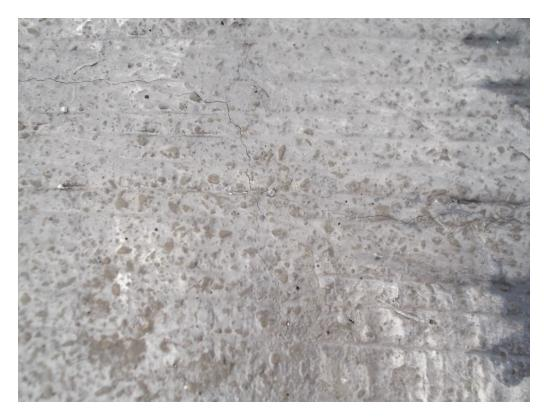
Fig. 7 – Cracks meeting at center of patch.
