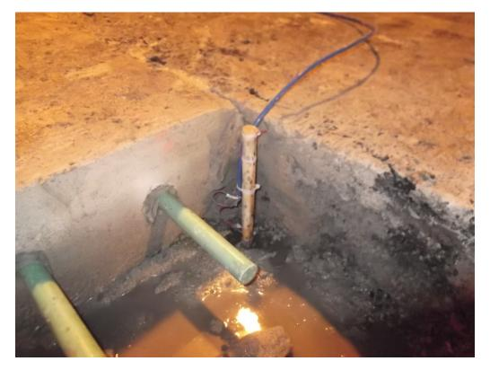
Fig. 28 – Layout of thermocouples at patch corner (patch 3).
