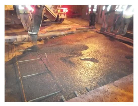
Fig. 29 – Concrete placement at patch 3.
