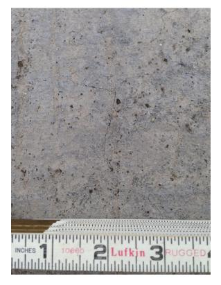
Fig. 18 – Cracking observed in nonaccelerated portion of patch 2.
