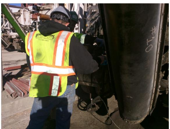
Figure 3 - Dispensing Accelerator for Calibration Procedure.
