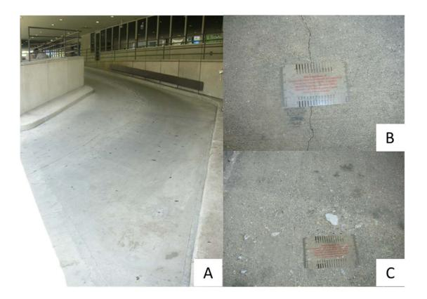
Figure 2-4 – (A) Emergency Entrance Ramp; (B) Cracking; (C) Scaling
