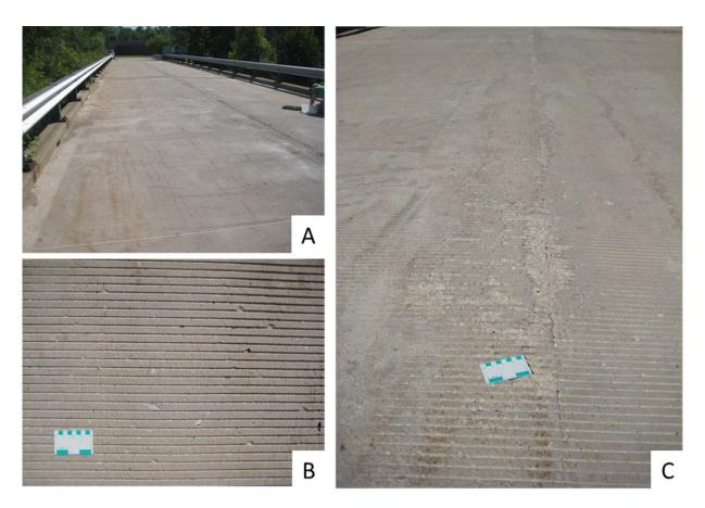
Figure 2-8 – (A), (B) Latex-Modified CAC Bridge Deck, (C) Abrasion Failure at Bridge Crown
