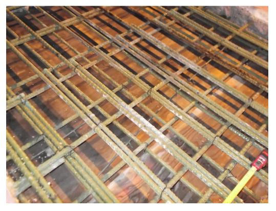
Fig. 4 – Layout of the reinforcement at the center of the patch.
