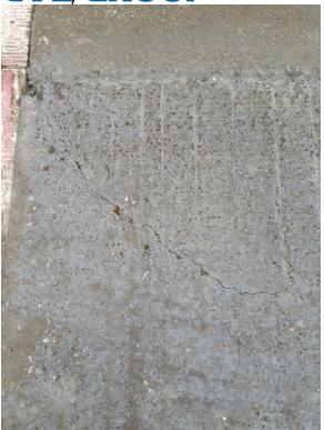
Fig. 20 – Cracking at interface between accelerated and non-accelerated portion of Patch 2.
