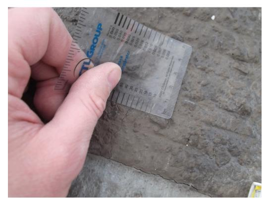
Fig. 8 – Longitudinal crack at south edge (0.25mm).
