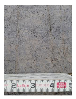
Fig. 19 – Cracking observed in nonaccelerated portion of Patch 2.
