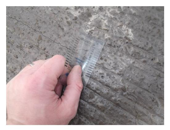
Fig. 9 – Transverse crack (0.50mm).
