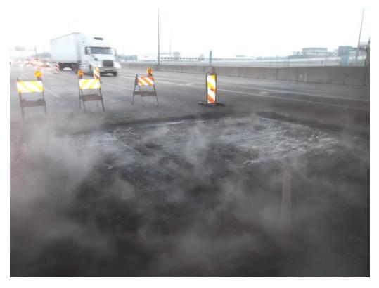
Fig. 32 – Finished patch 3 (after removal of plastic, before saw-cutting).
