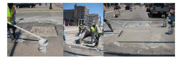
Figure 2-6 – Partial-Depth CAC Repair, Roosevelt Bridge, Chicago, IL
