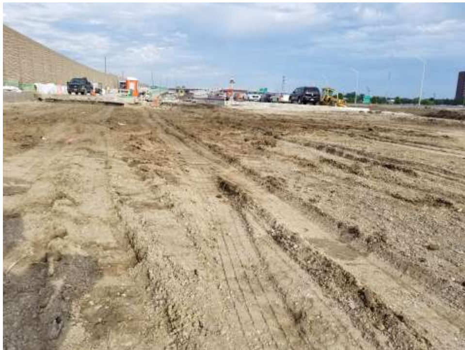
Figure 49. Pictures of subgrade during and after proof rolling near southwest corner of TS14
