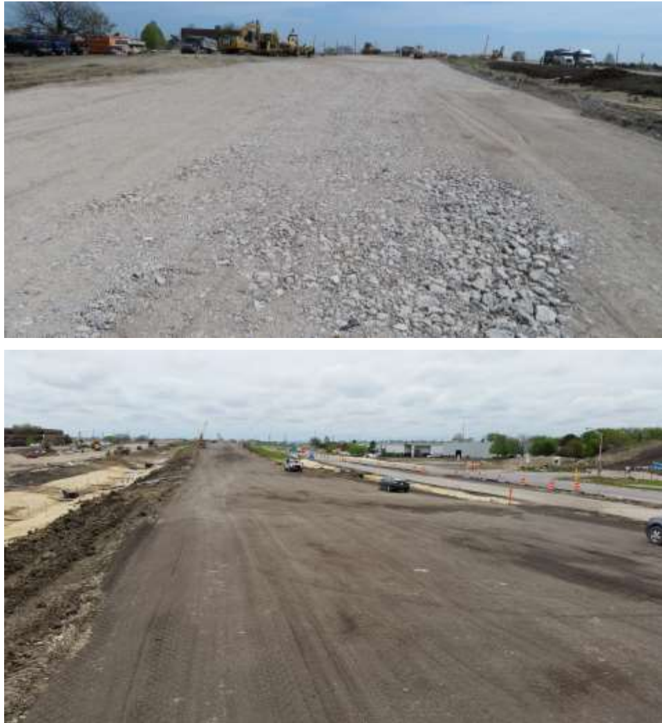
Figure 38. Pictures of CA6 capping material from PGE material from TS11 (middle-04/25/17) and CA6 material from TS12 (bottom-05/04/17)
