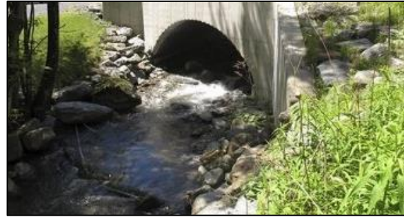
Figure 4 - Culvert on Crossett Brook, Danbury, CT. This is an example of downstream grade control that allows for fish passage. (AP photo).
