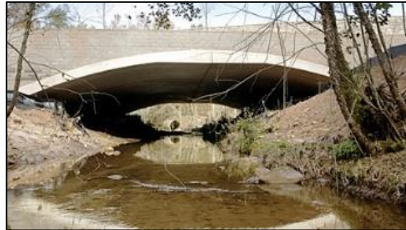
Figure 2 - Example of a structure that appears to span WOUS. Bebo pre-cast bridge. (pamonapipeproducts.com)
