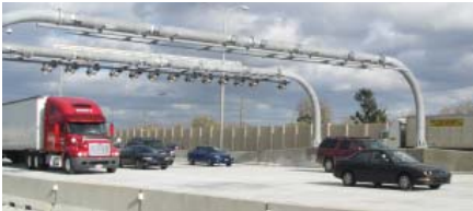
Open road tolling at Illinois Tollway's Irving Park Plaza.
