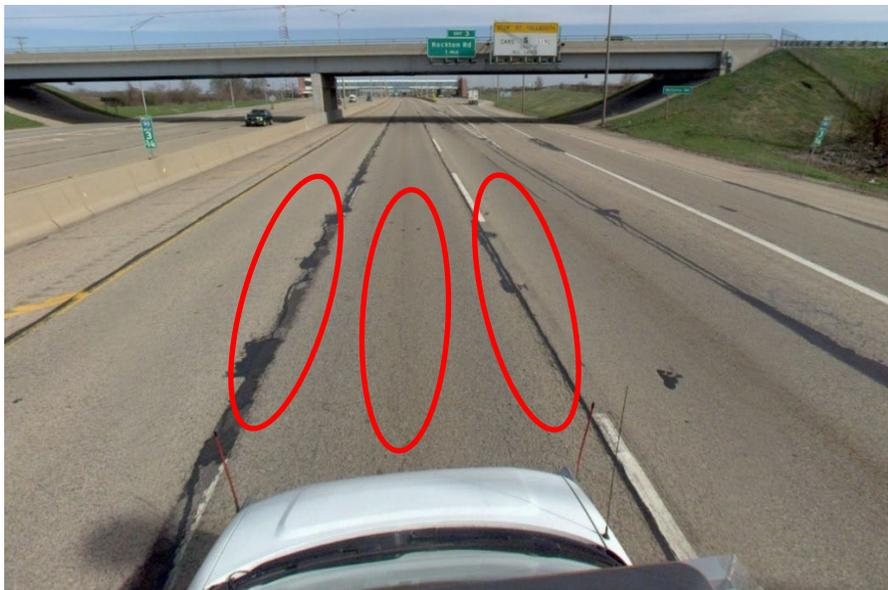
Figure 6-6. Longitudinal cracks that join the transverse cracks - I90-6.6 section
