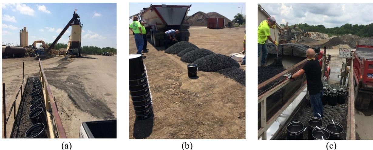
Figure 2-1. Sampling plant produced mixtures from different asphalt plants. a) Mix 1836, Wm Ch; b) Mix 1845, Curran, and; c) Mix 1807, Geneva.
