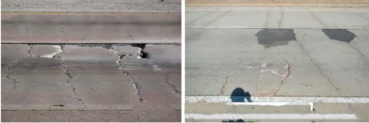
Figure 20. Punchout at CRC pavement (Jeon, Choi & Won, 2019).
