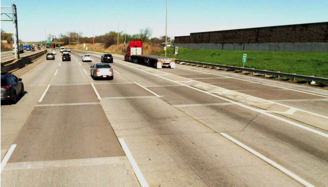
Figure 25. Example of rapid full-depth repair with precast concrete.
