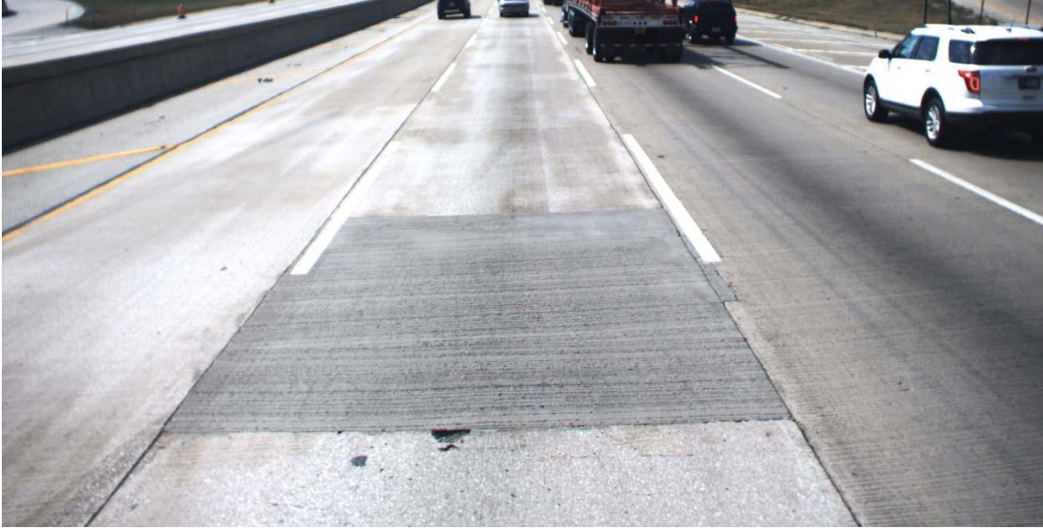
Figure 24. Example of full-depth patching of CRC pavement.
