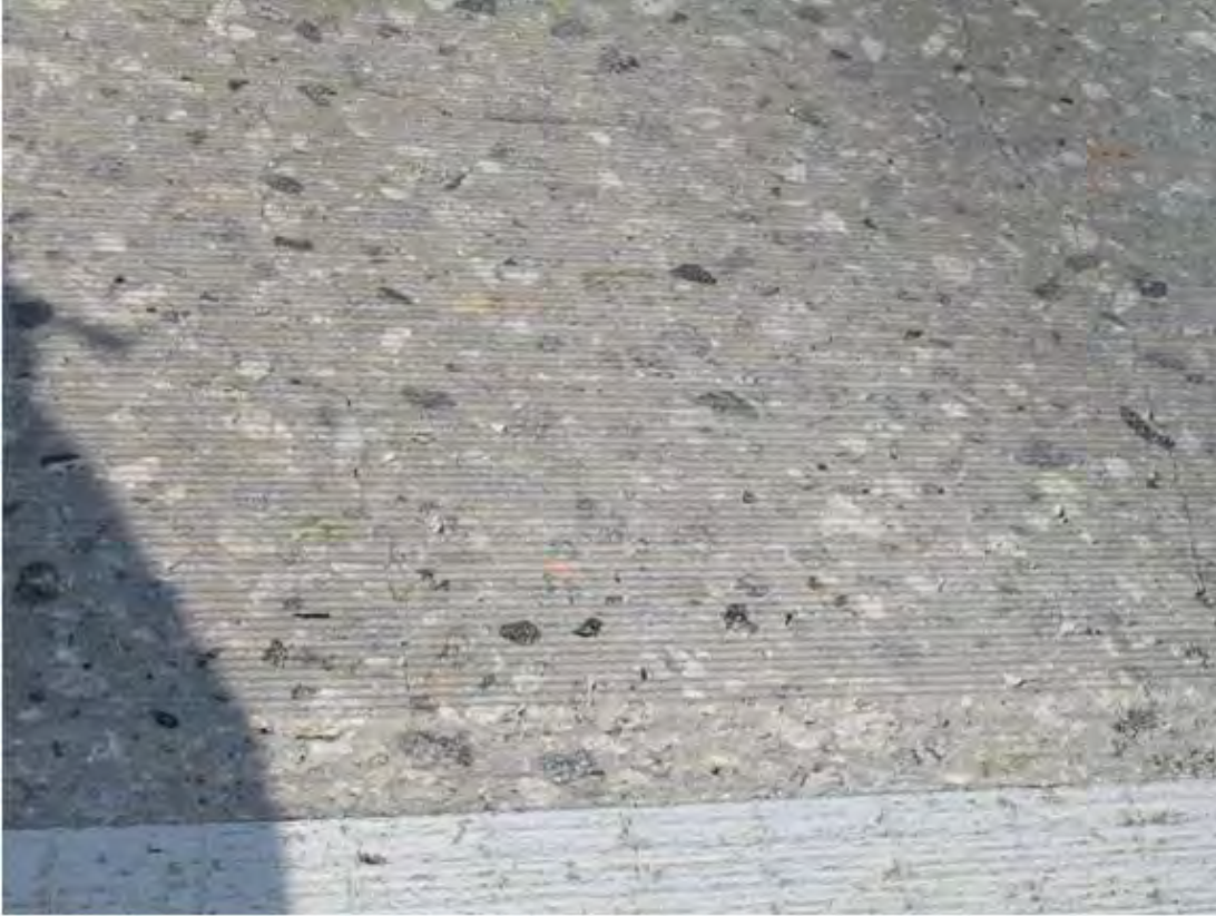
Figure 28. Diamond ground surface (TxDOT, 2019).
