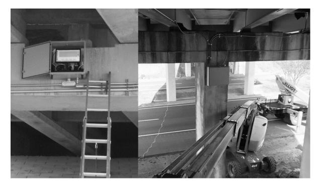
Fig.9 Typical NEMA enclosure and their locations in previous installations.
