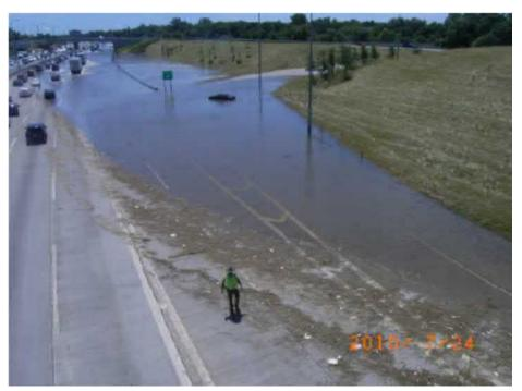
Figure 19: I-294 SB Flooding looking at Cermak Exit Ramp – debris on pavement shows HWL (Photo from EJM- Primera)
