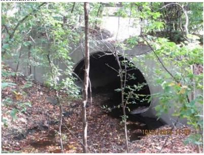
Figure 7: 11.6' (W) x 7.33' (H) Arch CMP Culvert under Creek Drive
