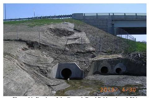
Figure 16: Erosion of the Cermak Road Bridge along I-294
