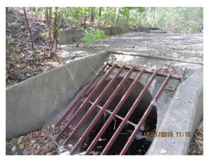
Figure 9: Concrete Grate Structure, downstream of Creek Drive
