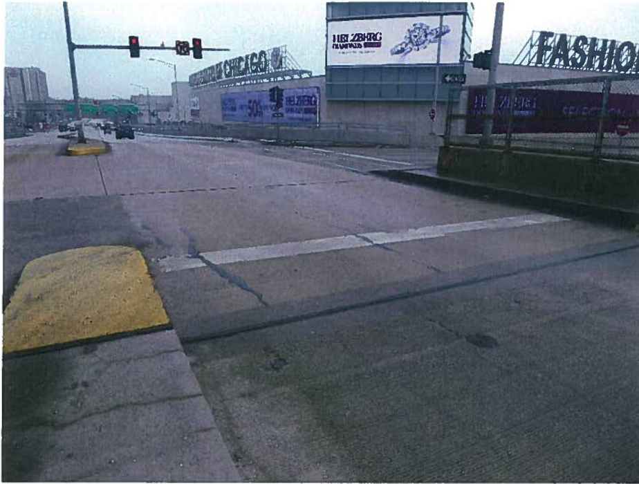
5 – East Approach Slab longitudinal cracking and deck spalling (Eastbound)
