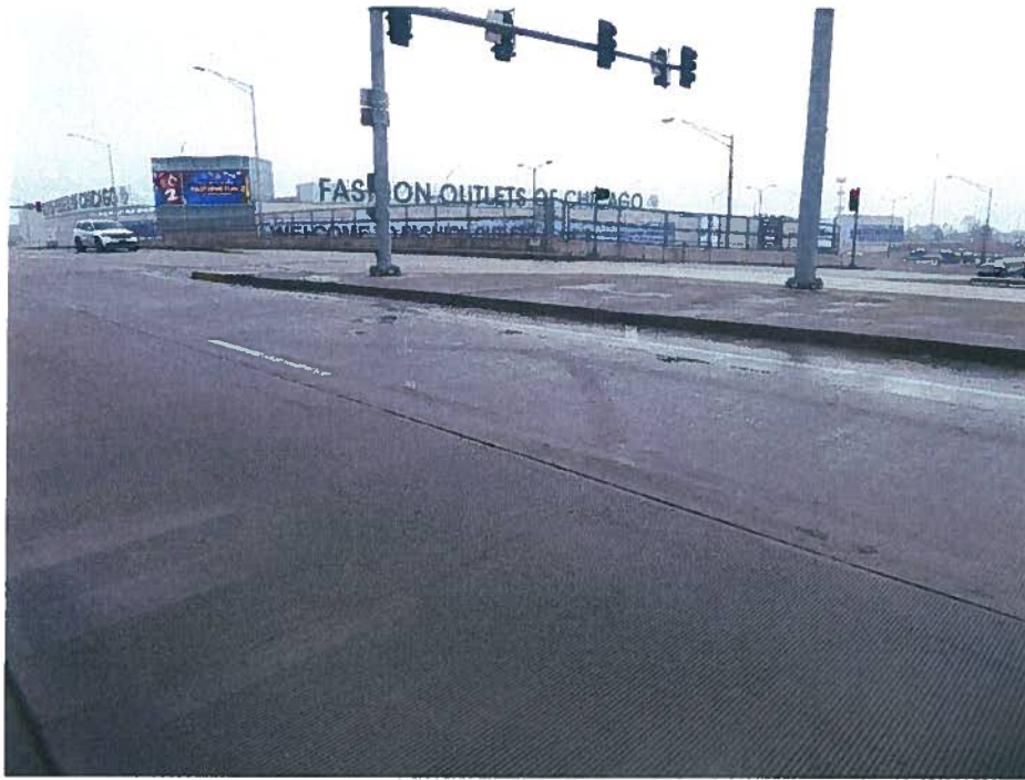
1 – West Approach Slab spalling and transverse cracking (Westbound)
