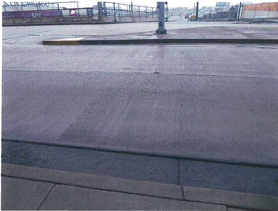
3 – West Approach Slab transverse cracking (Westbound)
