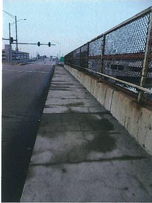
7 – North sidewalk cracking (Westbound)
