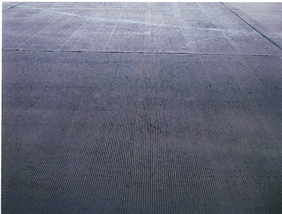
4 - East Approach Slab longitudinal/transverse cracking (Westbound)
