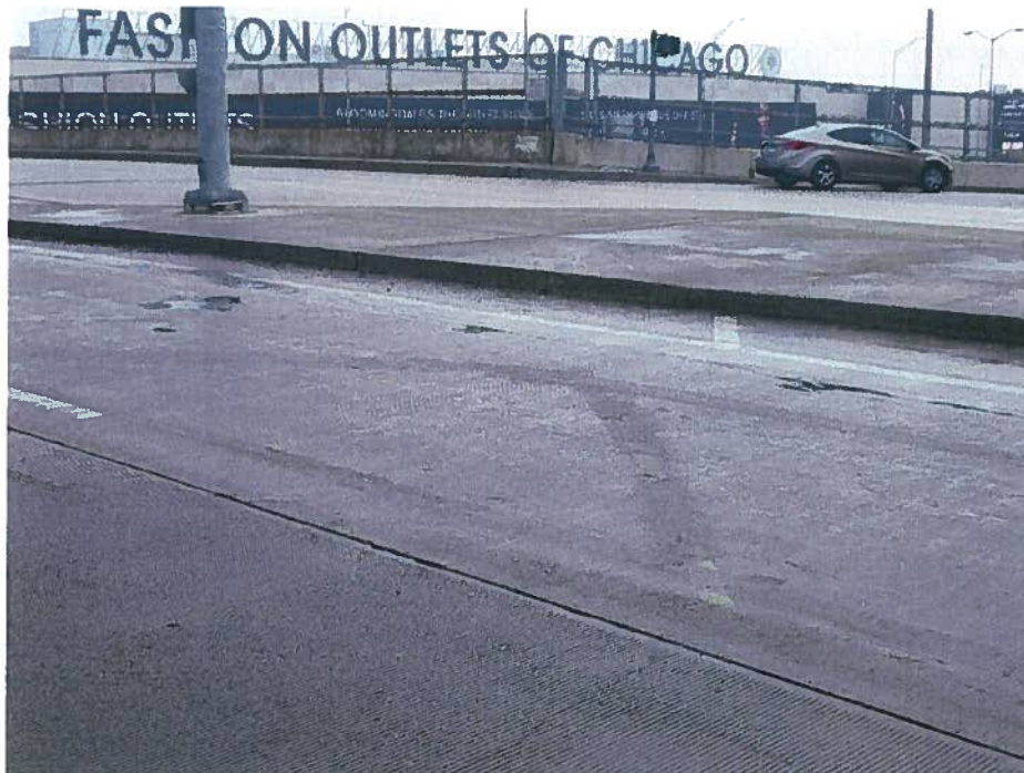
2 - West Approach Slab spalling (Westbound)
