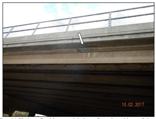
Photo 16: Waukegan Road, beam repair in the top flange, beam 1 in span 3 shown
