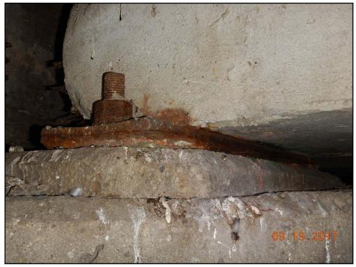
Photo 18: Waukegan Road, typical fixed bearing with rust
