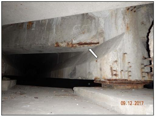
Photo 15: Waukegan Road, typical spalled diaphragm
