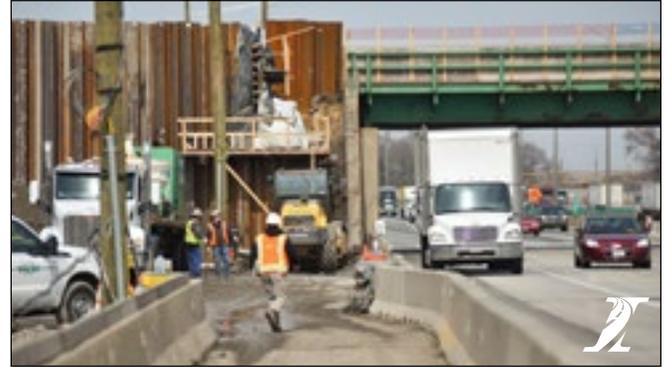
To build the shoefly bridge, construction crews working in roadside staging areas will assemble bridge segments from steel beams while they are safely away from traffic. Using roadside staging areas also allows them to work during the day without interruptions and near ground level in a safer environment.
