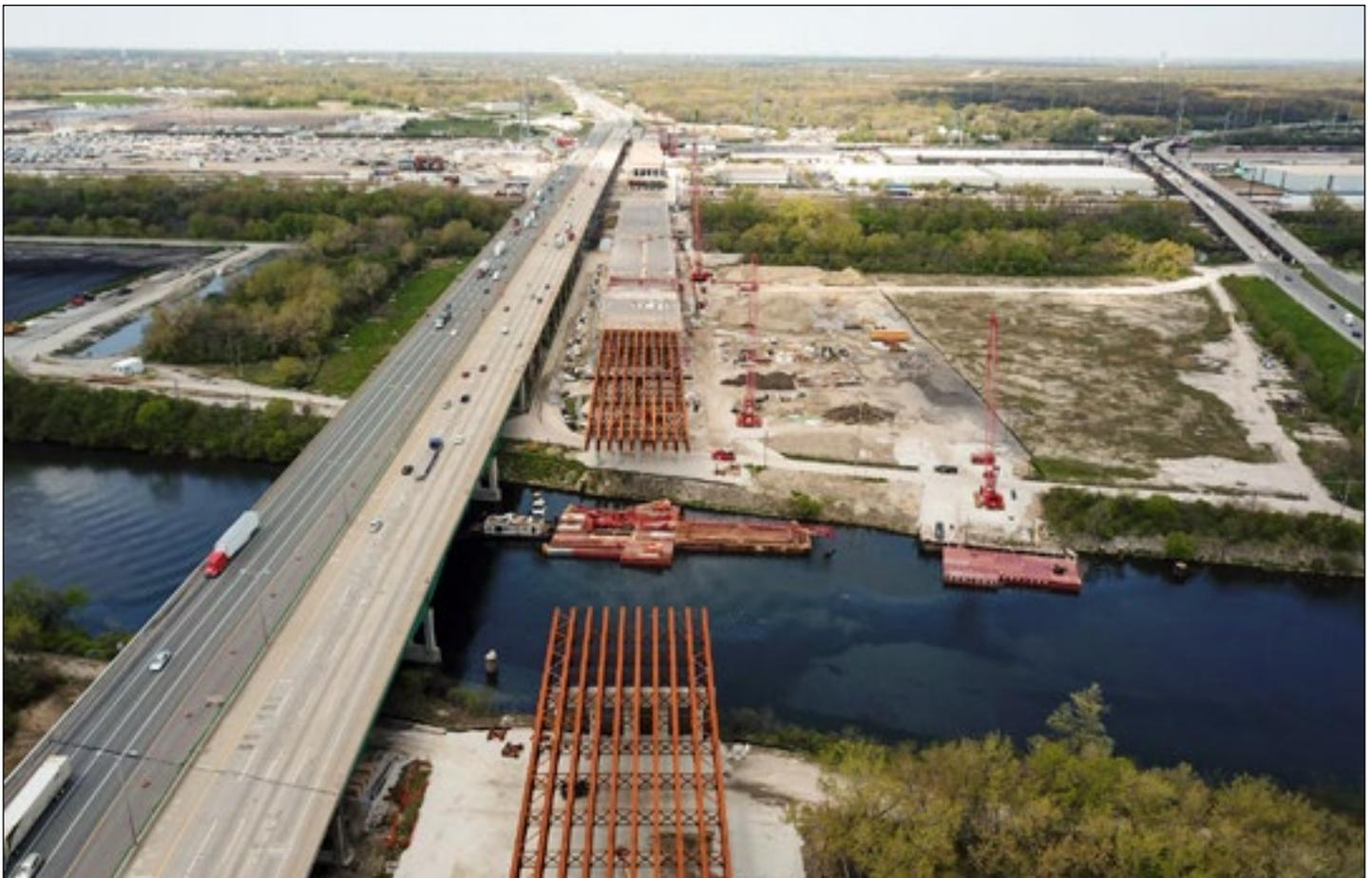
Using those techniques will significantly reduce the impact on Tollway customers by requiring few lane closures on I-294 while the bypass or "shoefly" bridge is being installed above it.
