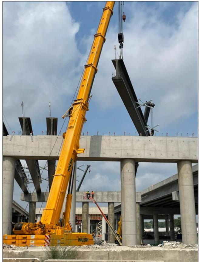
will be installed over the County Forest Preserve property and the Chicago Sanitary & Ship Canal. Each of the steel beam segments will measure between 86 and 120 inches tall and between 39 and 234 feet long.
