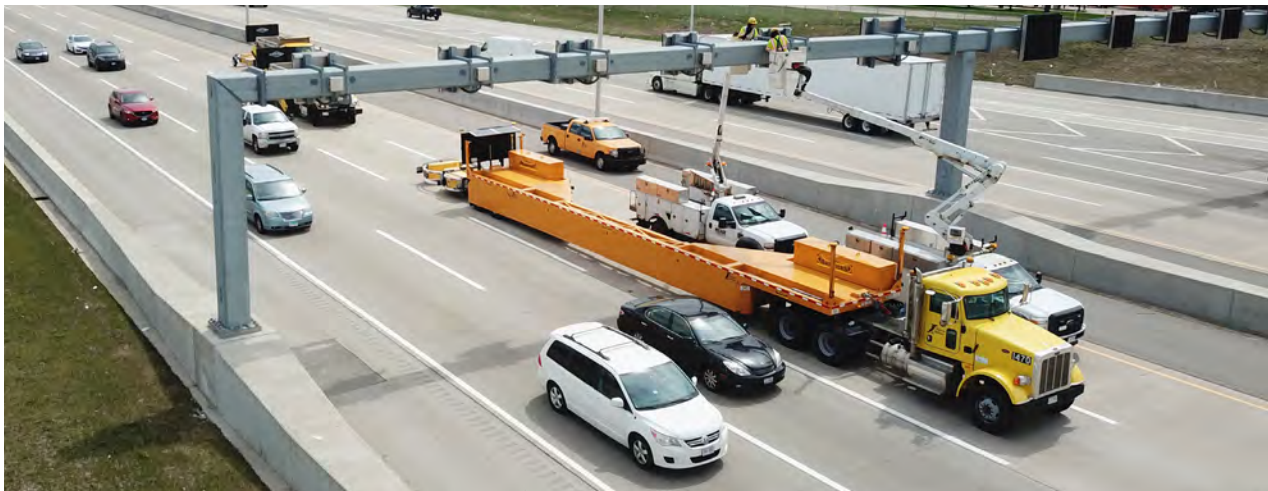
Gantry repair on WB I-90
