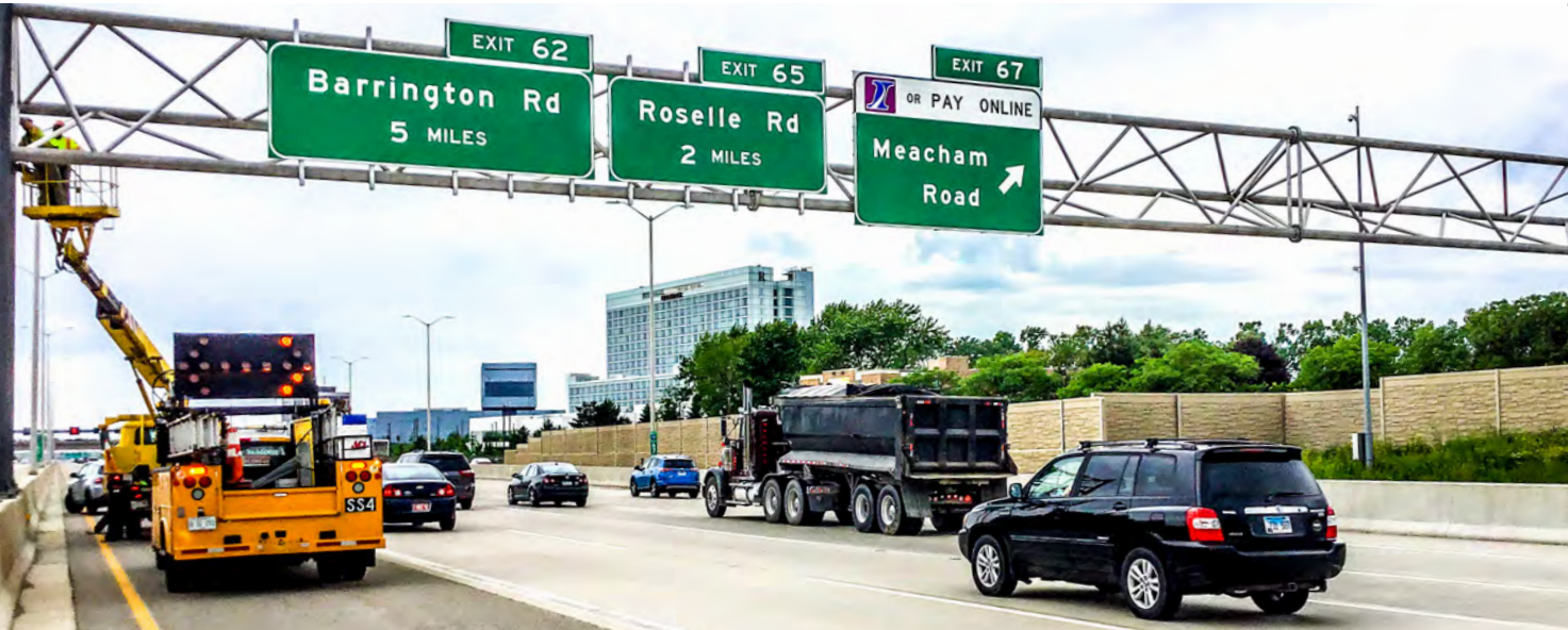
Sign structure inspection on I-90 Westbound
