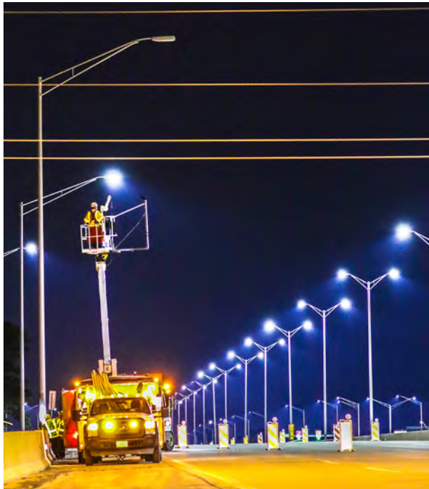
LED light pole retrofit on EB I-88
