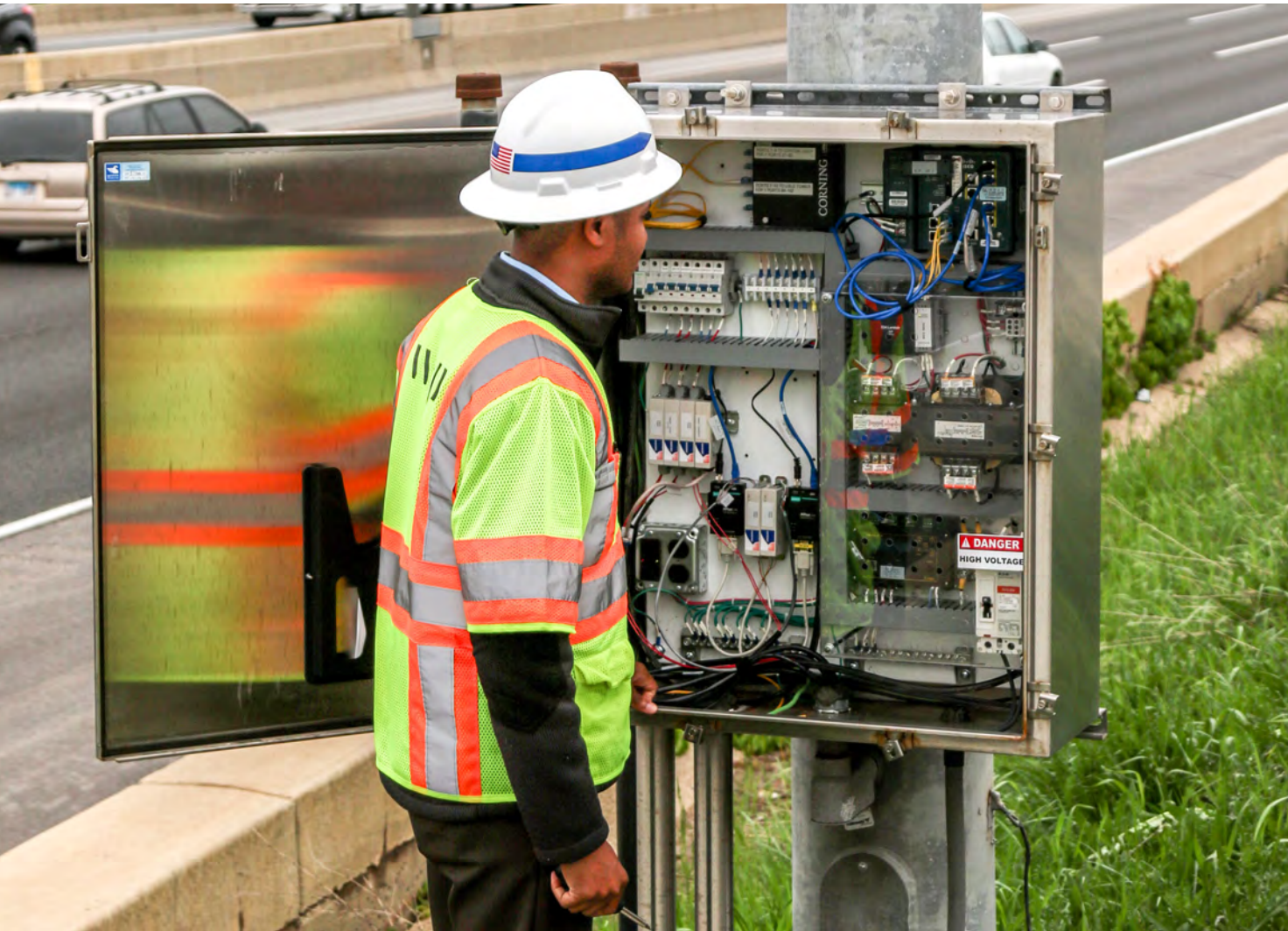
ITS Cabinet Inspection between I-88 and I-355
