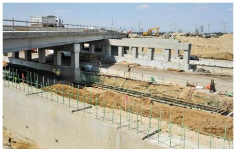
Jane Addams Memorial (I-90)/Illinois Route 47 Interchange construction - A pier foundation is formed for the Illinois Route 47 bridge (5/1/2013)
