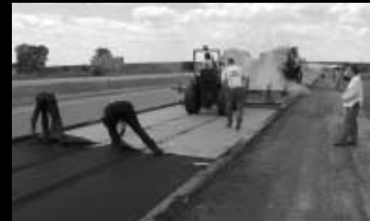
Northwest Tollway resurfacing project
